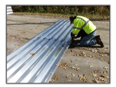
Structural Plate bridges and culverts can be cost effective alternatives to traditional bridge replacements depending on the site.
